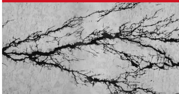
Fig. 8-2 Stress Corrosion Cracking Failure of 300 Series Stainless Steel
