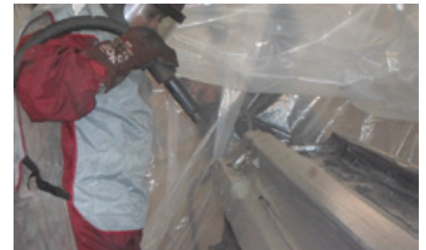
Shot peening technician working on a localized area of concern
